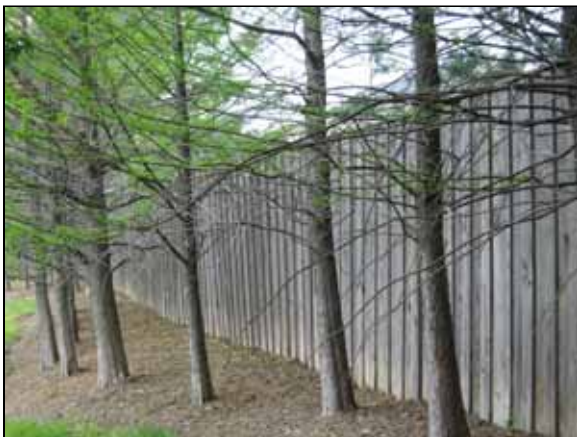
Photo #47. General view of the stockade fence installed along Walney Road.
