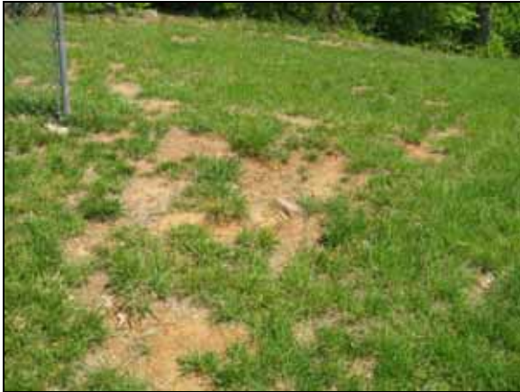
Photo #7. Common area does not have proper ground cover.
