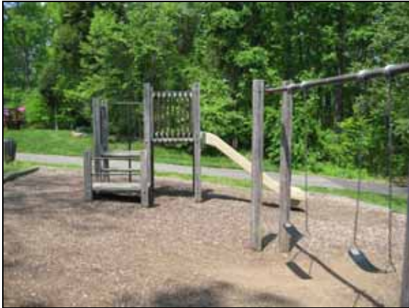
Photo #25. Gaston Tot Lot. Note lack of proper ground cover at the swing.
