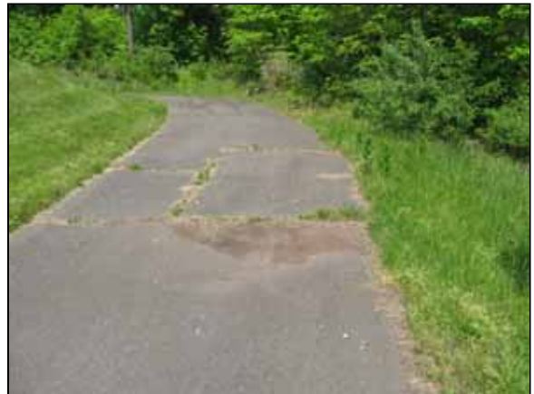
Photo #34. Deteriorated asphalt pavement, Tot Lot / SWM access road off of Gaston Street.
