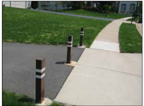
Photo #22. Metal bollards at the Tot Lot / SWM access road.
