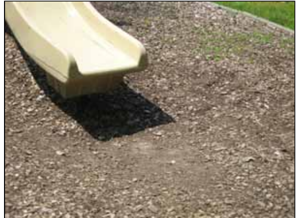
Photo #32. Inadequate resilient ground cover, Gaston Tot Lot.
