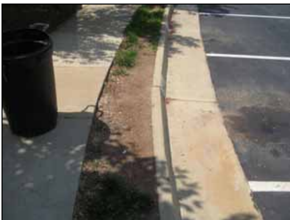
Photo #17. Area between sidewalk and curb & gutter without proper ground cover, Penny Tree Place.
