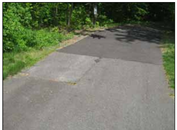
Photo #24. Tot Lot / SWM access road located off of Gaston Street.
