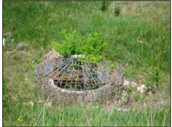
Photo #8. Storm water structure adjacent to the ball field.
