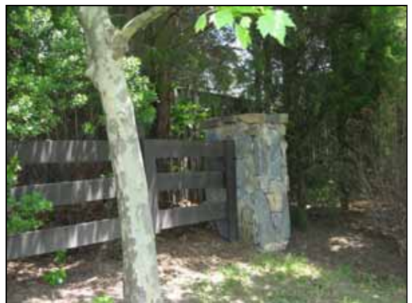
Photo #42. End of the three rail fence into a stone pier, Walney Road.
