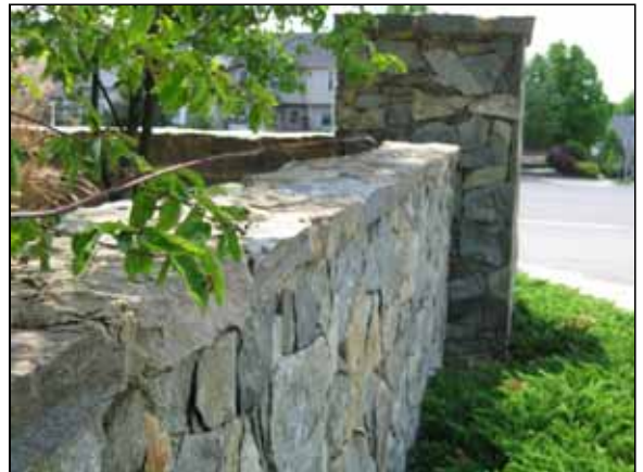
Photo #40. General view of the entrance feature.
