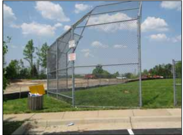
Photo #2. Backstop. Note construction in progress on the adjacent property.
