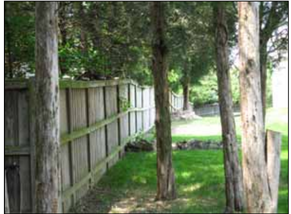
Photo #44. Stockade fencing installed along Walney Road. Note organic growth on the fence.
